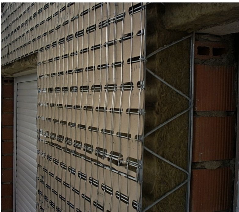
Stucanet system detail
